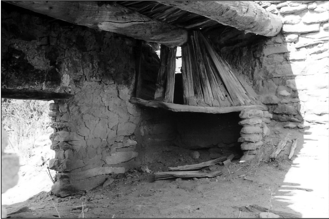
Figure 12.3 Hooded fireplace at Frances Canyon Pueblito. Viga-and-latilla roof construction also visible.
